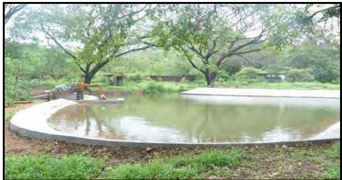
Water Harvesting Project at Colony
