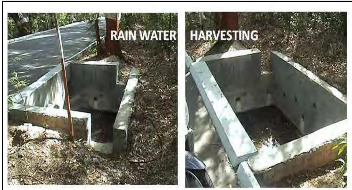
EXISTING RAIN WATER HARVESTING FACILITY
