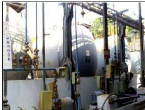
SOLVENT STORAGE TANK
