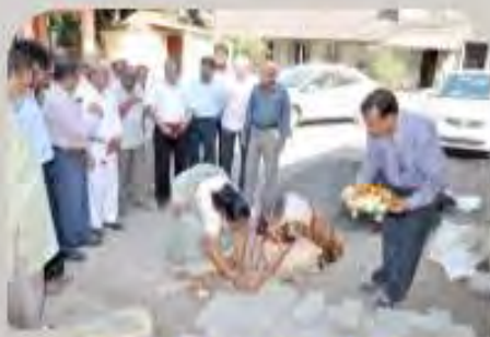
Paver block road
