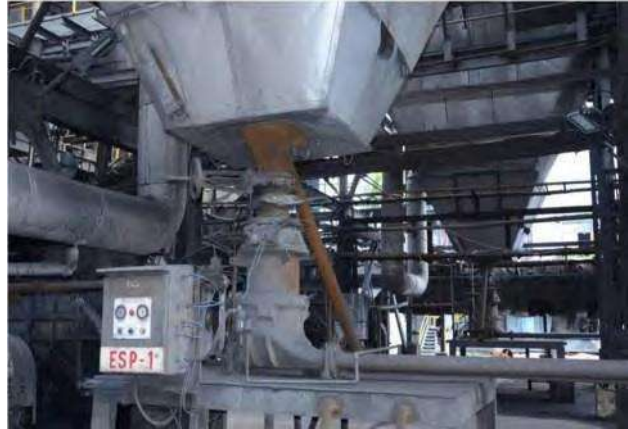
Dense phase pneumatic ash handling system
